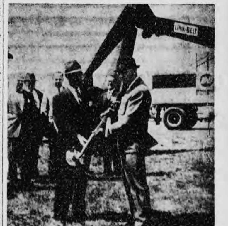
BREAK GROUND FOR ADDITION--Alonso G. Decker, Jr., president, and Robert D. Black, chairman of the board, Black and Decker Manufacturing Company, break ground for the 212,000 square foot addition at the Hampstead plant. The addition will provide 710,000 square feet of manufacturing space in the Carroll County facility.
