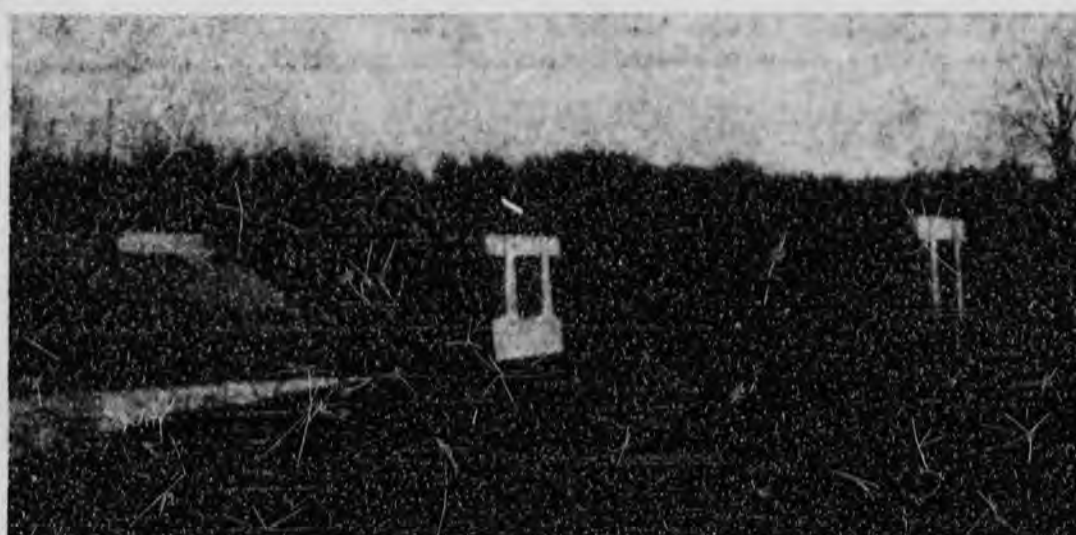
SUPERSTRUCTURE OF SYKESVILLE BRIDGE READY FOR CONSTRUCTION—The two piers and two abutments for the Sykesville by-pass bridge have been completed and work is expected to start soon on the superstructure. The by-pass bridge is on Route 32 over the South Branch of the Patuxent River and the Baltimore and Ohio Railroad in Carroll and Howard Counties. The State Roads Commission points out that the bridge when completed will be the first aluminum bridge of its kind in Maryland.
